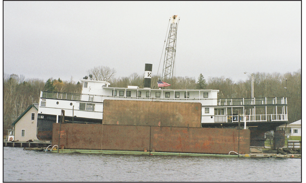
A side view of KATAHDIN inside the dry-dock showing the wing walls made from three pontoons. This is KATAHDIN's regular berth at Moosehead Marine Museum at Greenville. Following her re-launch she returned and was docked closer to the building with the dry-dock at her stern so it can be taken apart and shipped back to Rockland.
