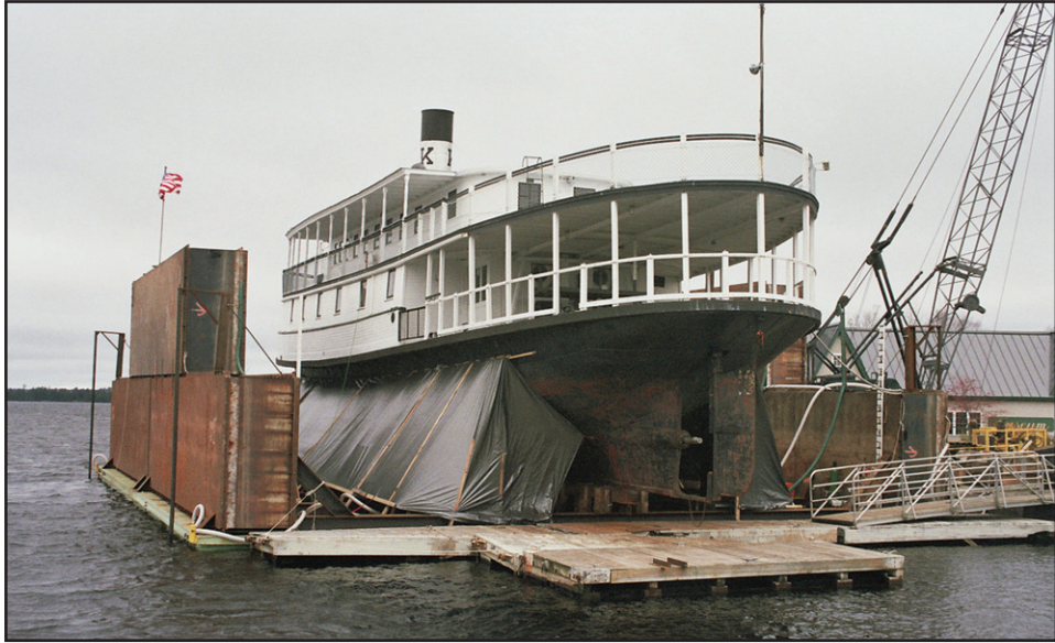
The stern view of the cruiser vessel KATAHDIN hauled out at Greenville. Repairs were made to her keel along with normal maintenance. Note the drydock, which was made with nine pontoon for the base, and three on each side for wing walls. Repairs were complete and she was re-launched 28 November.
