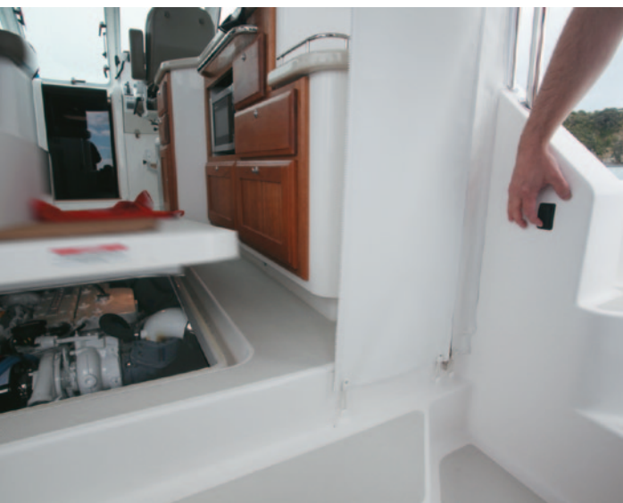
THE HELM DECK, INCLUDING THE PORT SIDE DINETTE, LIFTS HYDRAULICALLY TO EXPOSE THE YACHT'S MECHANICAL SYSTEMS BELOW.
